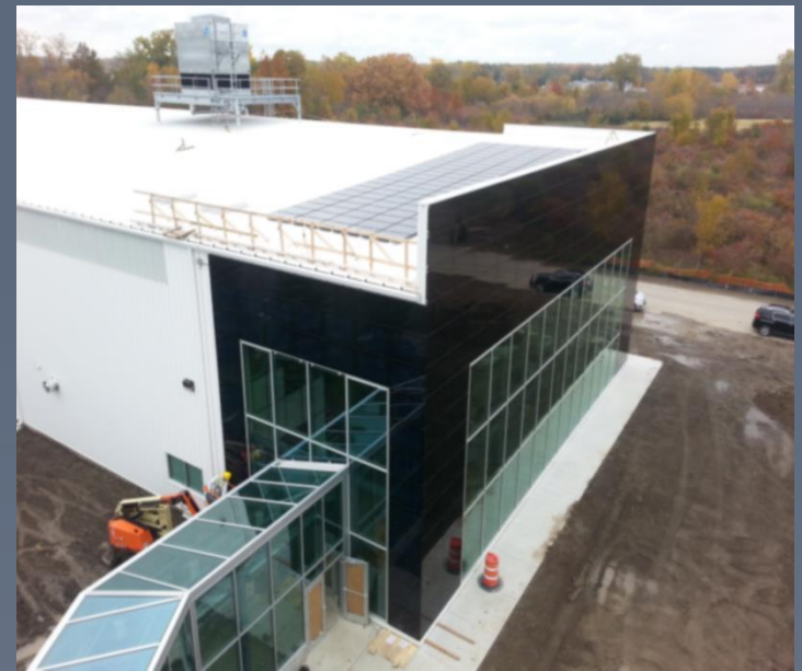
Architectural PV Glass Plus Rooftop PV
