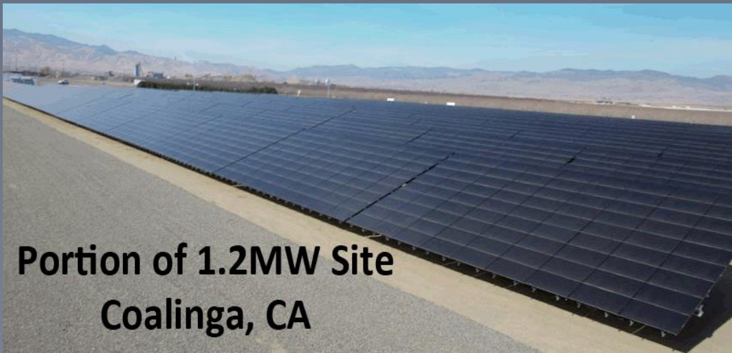
81-Module Block Design using CIS Thin Film Modules
