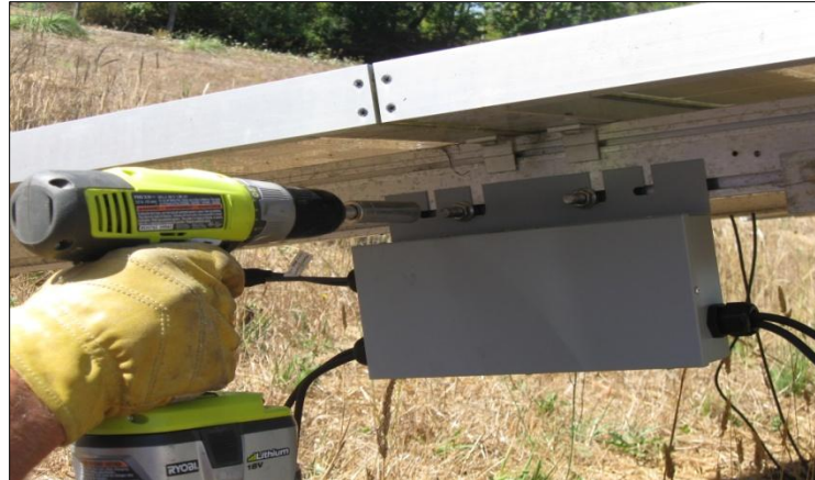
Figure 2. Mounting the vBoost to PV Array
